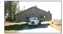
b. **Elevate:** If you don't have a high velocity flood hazard and you will receive a warning, the next safest alternative is to (3) elevate the building above the expected flood level. Buildings with crawlspaces in low velocity areas are the easiest to elevate. The steps are explained in a <u>brochure</u> from the International Association of Structural Movers and in FEMA's guide, <u>Above the Flood: Elevating Your Flood-Prone House (P-347).</u>
