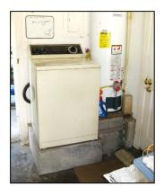
g. **Elevate your utilities:** Heating, air conditioning and electricity are vital utilities to make a building livable. If they are knocked out, it will delay repairing, rebuilding and reoccupying. One way to protect these utilities is to elevate them above the flood level, as in the example, below. Don't forget to elevate electrical outlets, too.
