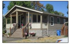
The end result is an open foundation or a higher crawlspace that allows floodwaters to flow under the first floor. Most <u>grant programs</u> that fund relocation can also help fund elevation projects. Raising the lowest floor above the base flood elevation may also lower flood insurance premiums.
