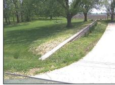
Do not backfill against your crawlspace wall because that may block the openings (see the next section). Also, if your crawlspace floor ends up below the fill level on all sides, it could result in higher flood insurance premiums.
