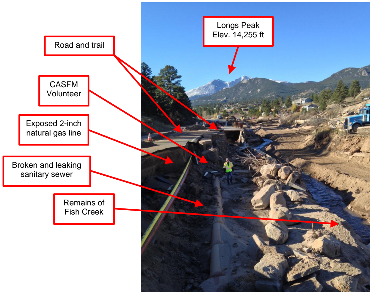
Figure 5. A view of public infrastructure heavily damaged along Fish Creek in Estes Park during a CASFM volunteer effort to collect high water mark information (Varrella 2013).
