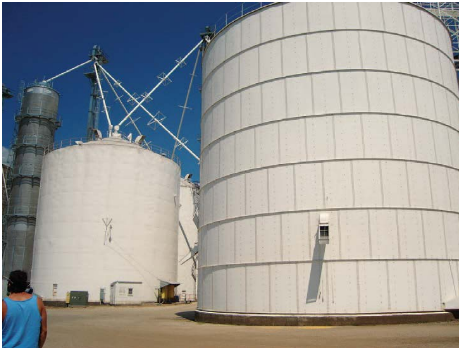
Figure 5. Bolted silos like the one on the right were prone to seepage during the 2008 Midwest floods and consequently contents were lost. Welded silos like the one on the left did not experience seepage. [Source: FEMA P-765, Midwest Floods of Iowa and Wisconsin. http://www.fema.gov/media-library-data/20130726-1722-25045-0903/fema_p_765.pdf ]
