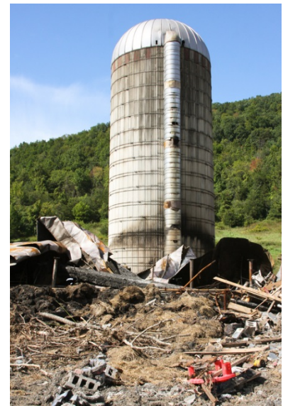
Figure 6. When hay inside this flooded silo became wet and hot, it spontaneously combusted. [FEMA, http://www.fema.gov/media-library/assets/images/62255 ]
