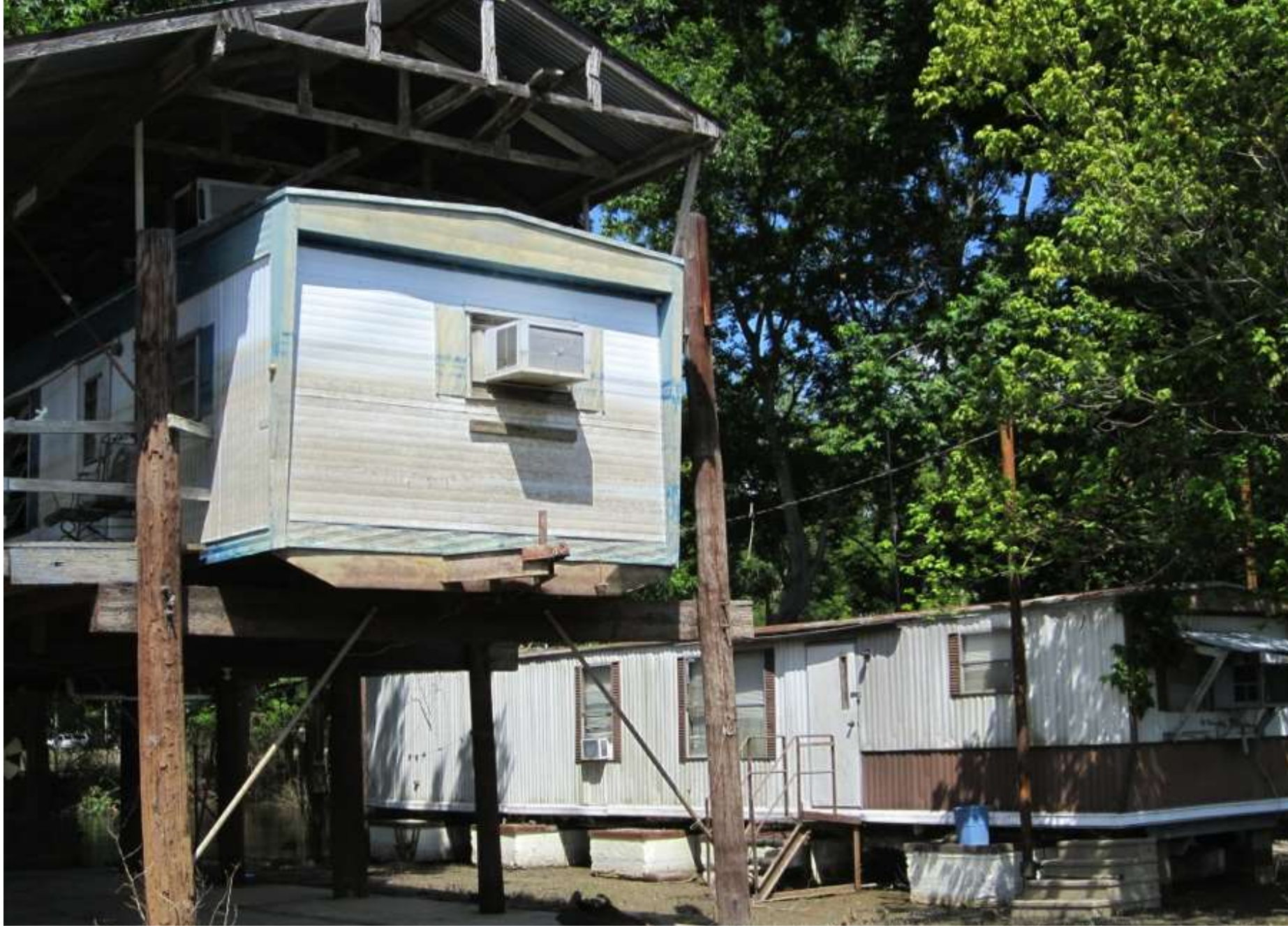
Extensive damage to elevated home on left. Undamaged amphibious home on right.
