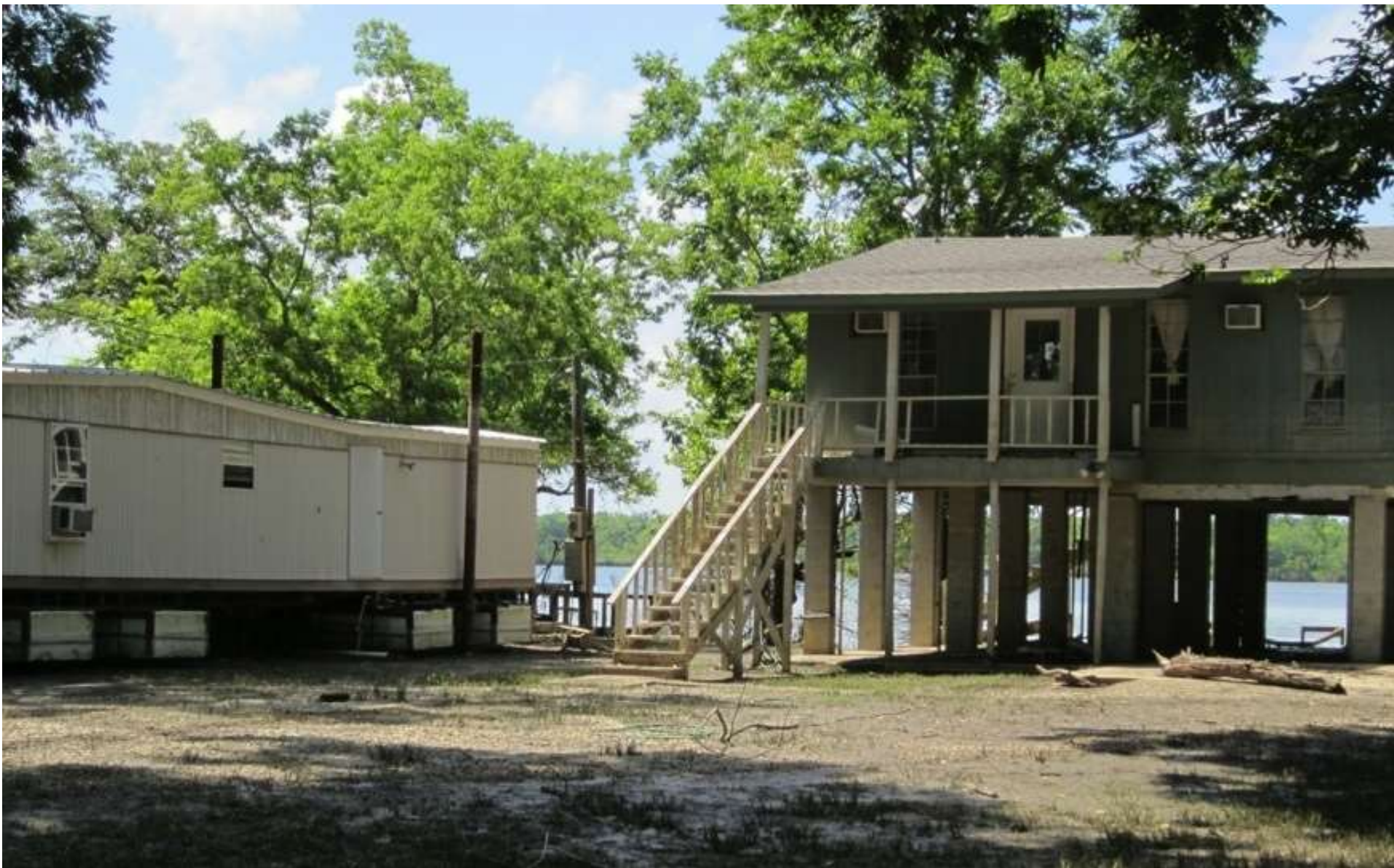
Undamaged amphibious home on left. Elevated house on right is extensively damaged.
